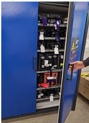
Figure 8 Safety storage cabinets for waste batteries (at Cleantron facility)
